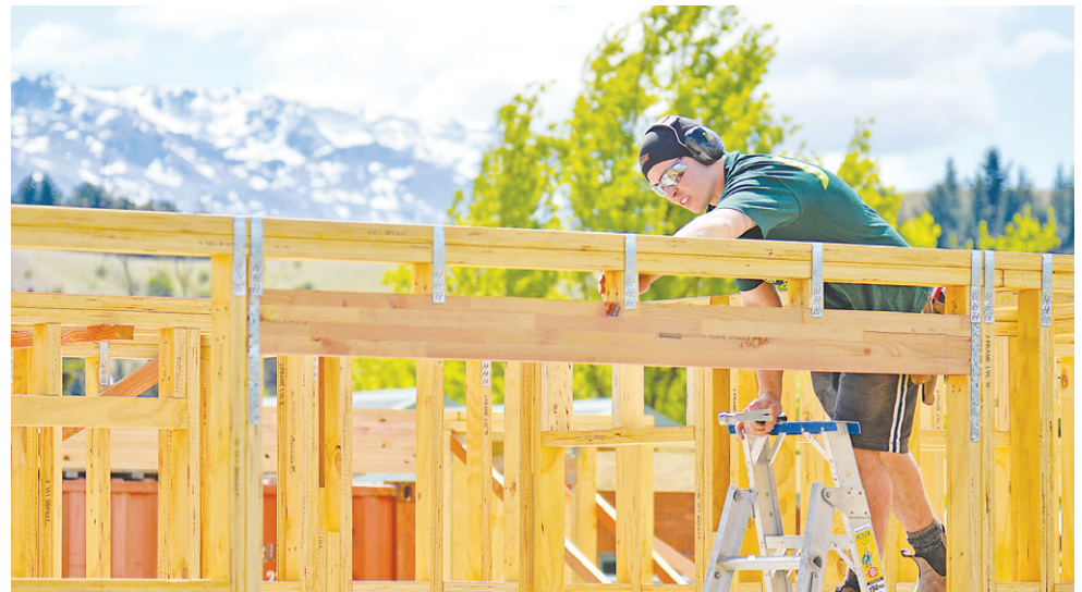
JNL's J frame timber being used in New Zealand construction.
