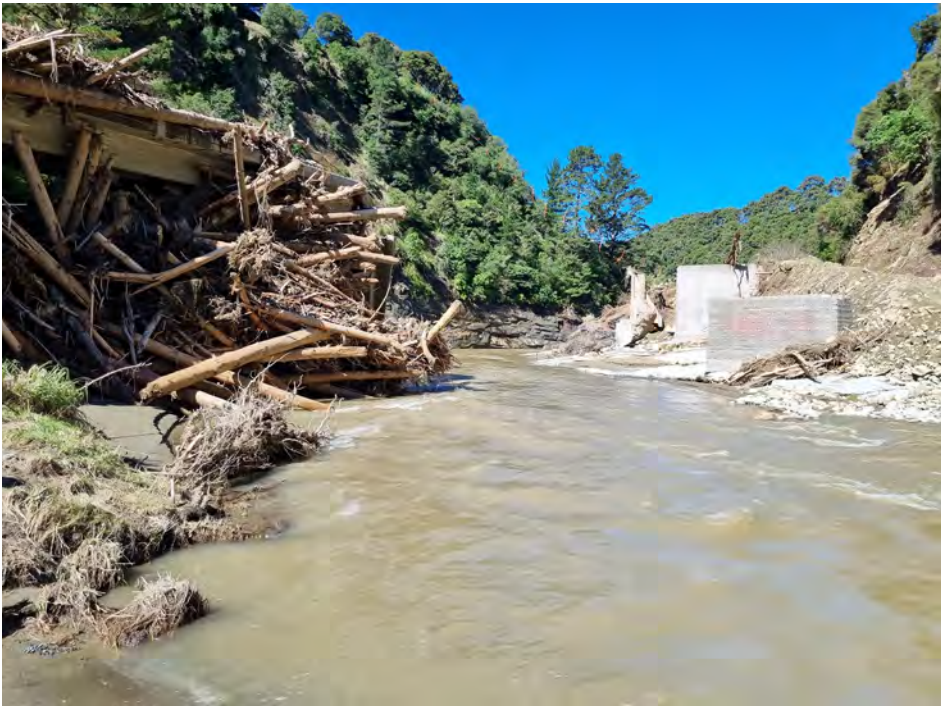
Figure 5: Broken State Highway 2 at Waikare
