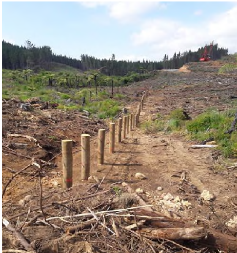
An example of a newly constructed trap using wooden posts. While also capable of trapping mobilised residues, its main design feature is to drive the residues from the main flow path onto the embankment where it can settle.
