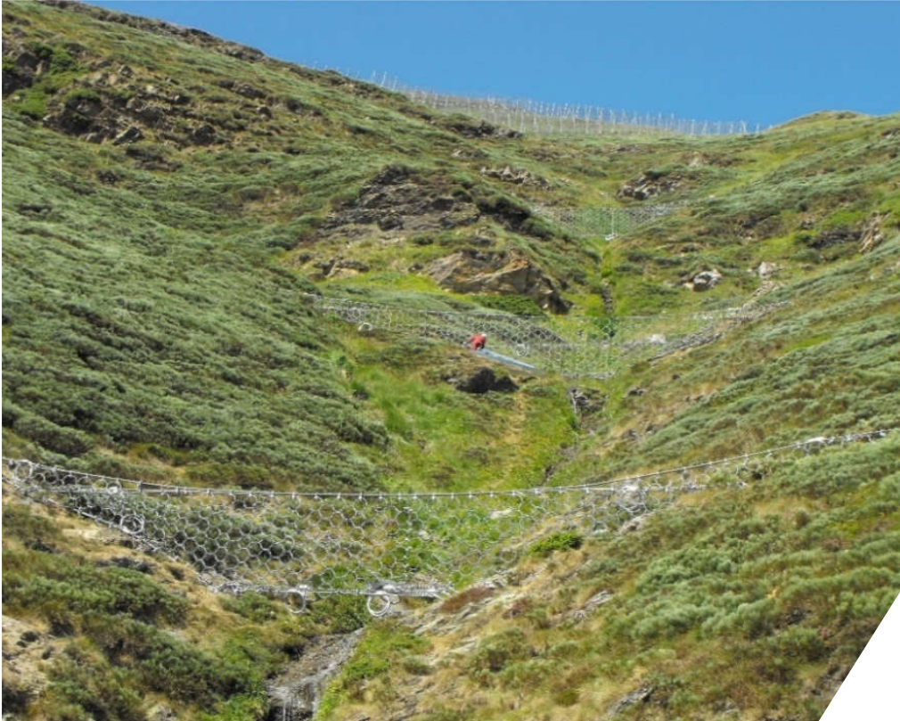
Figure 3 - Three debris barriers systems installed in Switzerland with low visual impact
